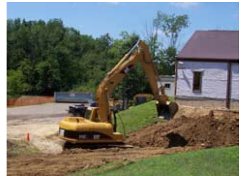
Excavating crews began preparing the foundation for the secure parking area and addition on July 25, 2006.
