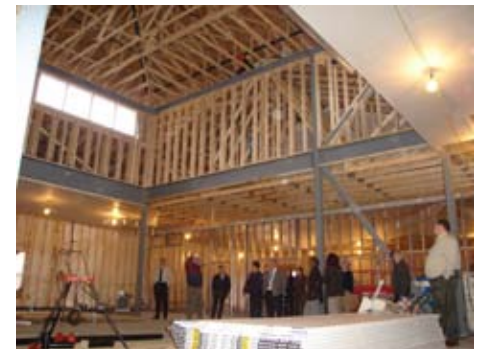
This picture shows the steel structure and wood framing that will become office space and the education/training wing.
