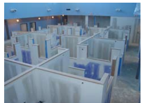
Same area as above nearing completion. Redesigned cubicles allow for personalized workspace and access to supervisor offices.
